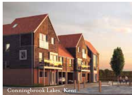
Conningbrook Lakes, Kent
