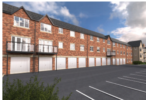
PARKING, GARAGING AND STORAGE
